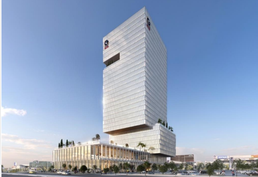
G CITY OFFICE TOWER – 60,000 SQM
