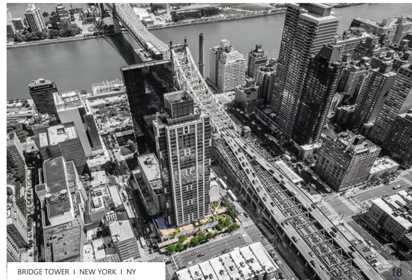
BRIDGE TOWER | NEW YORK | NY
