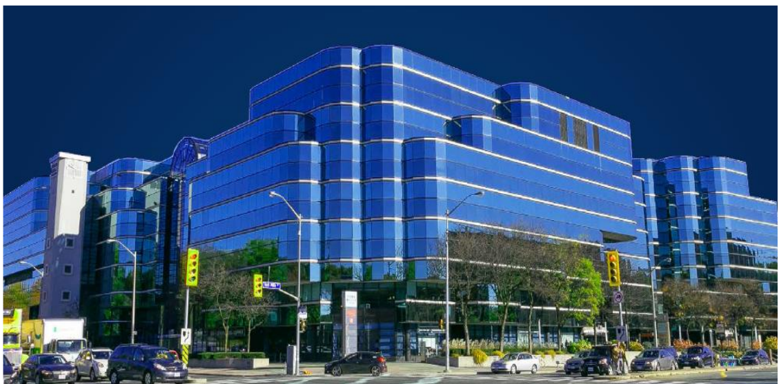
YORK MILLS CENTRE | TORONTO | CANADA
